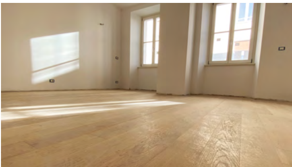
Historic building renovation Trieste, Italy
